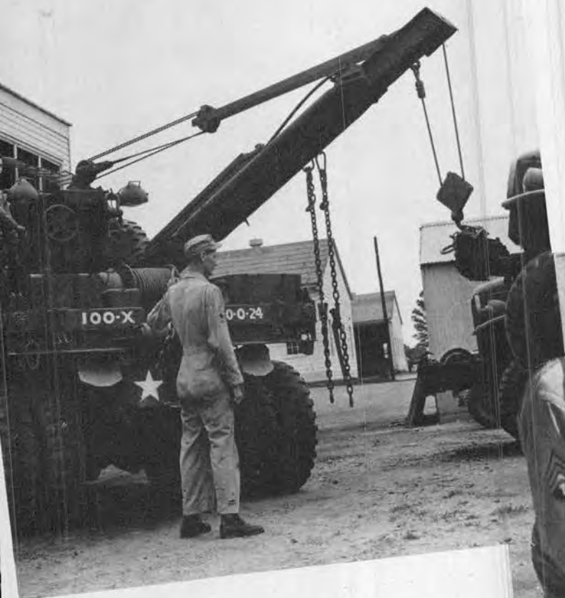
Wrecker of Ordnance Company tows immobile trucks to the shop for repairs.
