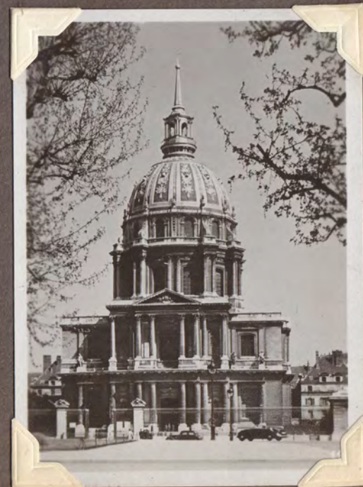
The Dome of the Invalid
