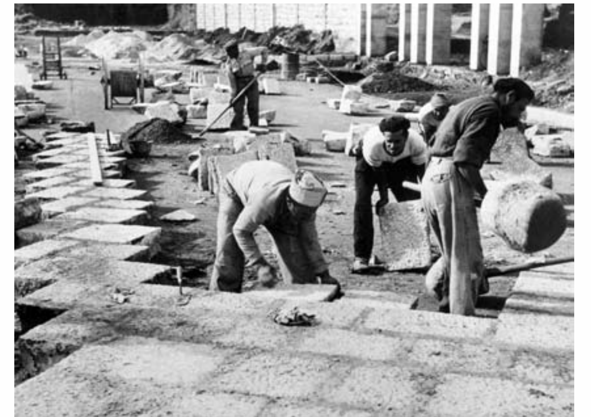
Building a road in Palermo, Italy.
