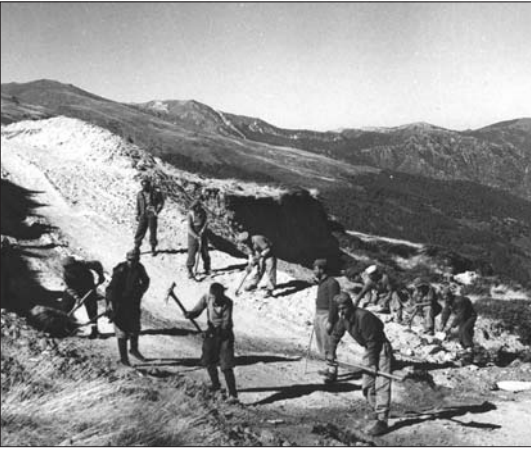
Greek Army engineers repair a road.
