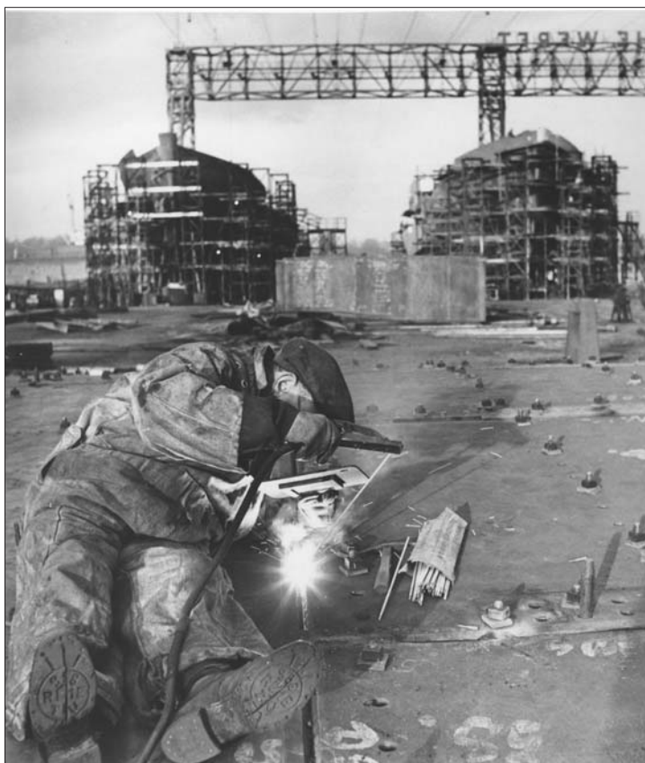
At the Deutsche Werft Shipyard in Hamburg, a shipyard worker shades his eyes as he uses a welding tool. In the background are two new ships under construction.
