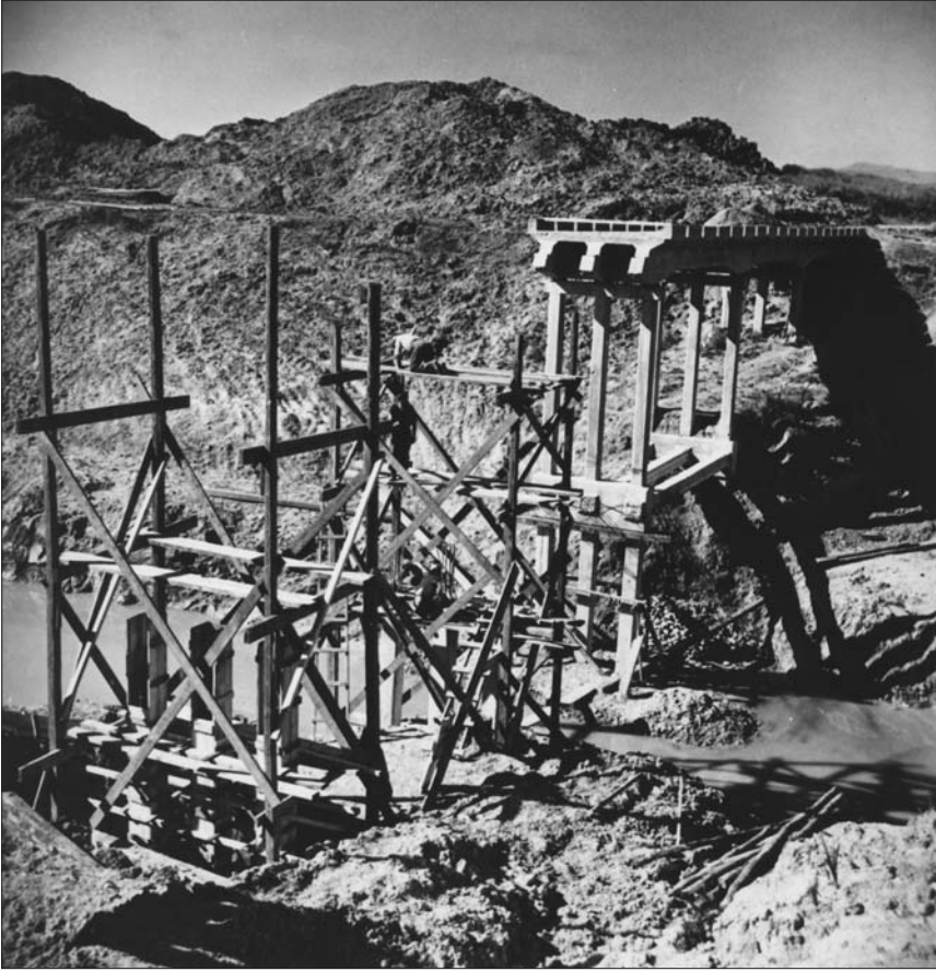
Workmen repair a bombed bridge in Macedonia.
